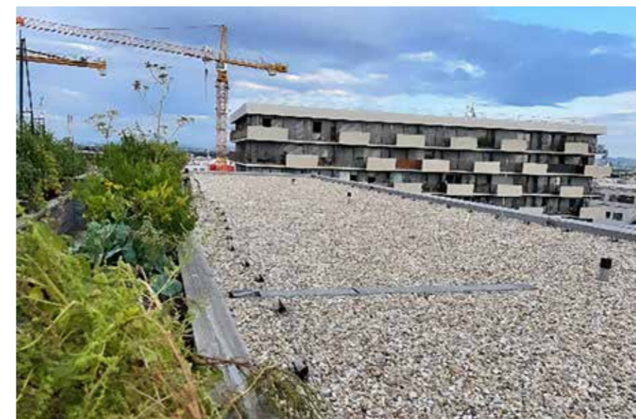
Obrázok 42 Udržujte voľné plochy pre fotovoltaiku, Co-living Seeparq, POS architektken Figure 42 Keep areas free for photovoltaics, Co-living Seeparq, POS architecten
