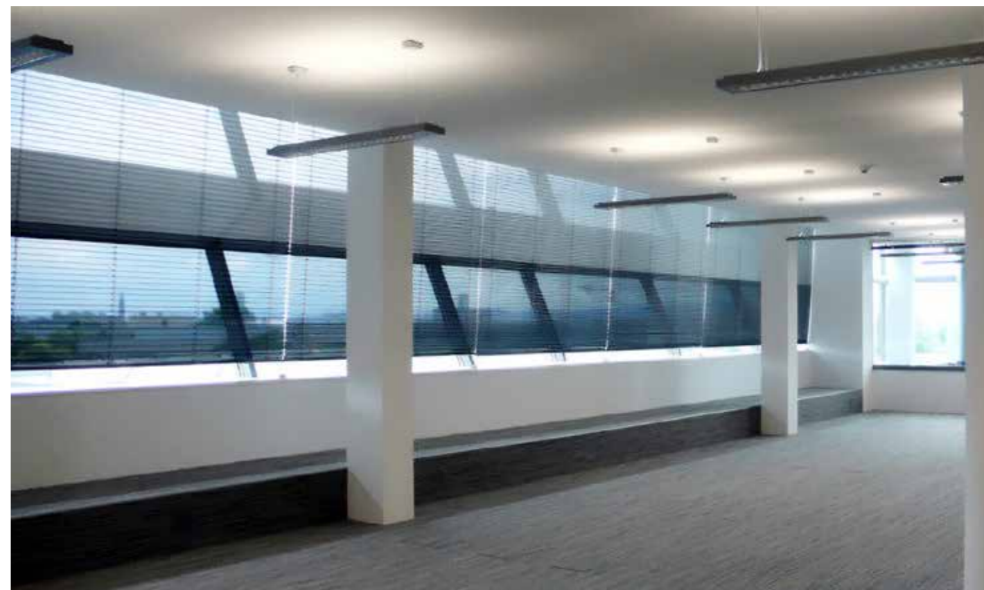
Obrázok 30 Transparentná perforovaná slnečná clona, ENERGYbase, POS architektken Figure 30 Perforated sunshade with transparency, ENERGYbase, POS architektken
